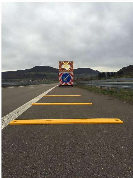
Figure 19: Portable rumble strips on hard shoulder
