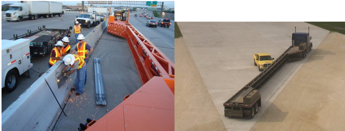
Figure 27: Work behind mobile barrier (left) and crash test of system (right)
