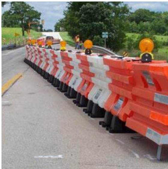
Figure 28: Water-filled portable vehicle restraint systems
